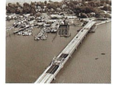
RON TURNER City Island Bridge - From the Air, 1979
